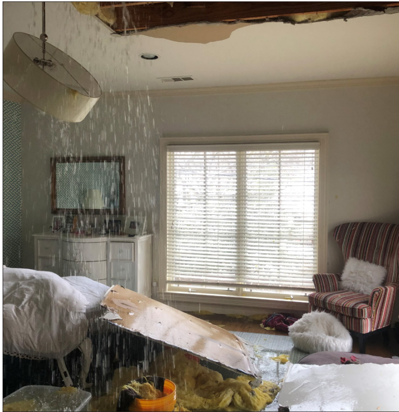
WHEN IT RAINS Drenched in water leaking from the ceiling, eighth-grader George Hoverman's sister's room sustained significant structural damage after a frozen pipe burst. Luckily, the Hovermans salvaged smaller personal belongings.
