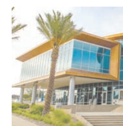
Photo Courtesy of SC
