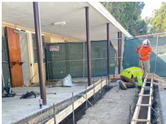
A new ramp is being installed in the library complex.
