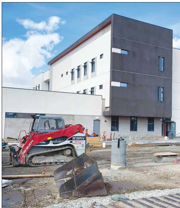
CAMPUS / A bond approved by voters in 2012 was used to construct the Central Mall and Johnson Student Center.
